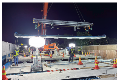
Installation status of new floor slabs
