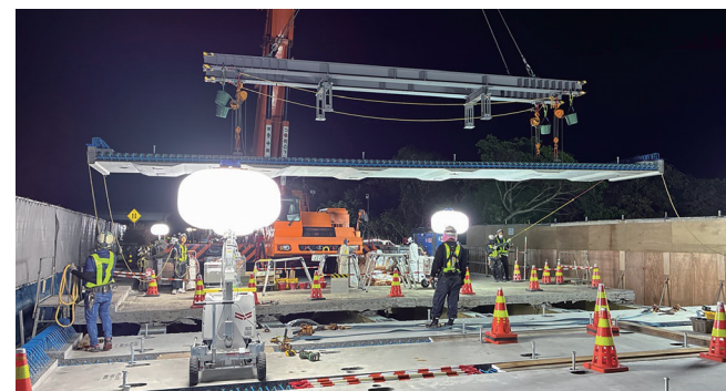
Installation status of new floor slabs
